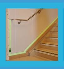
Using a high quality, fire retardant photoluminescent insert, our LLL system will continue to highlight a safe route in the event of power failure, fire or smoke ingress.
